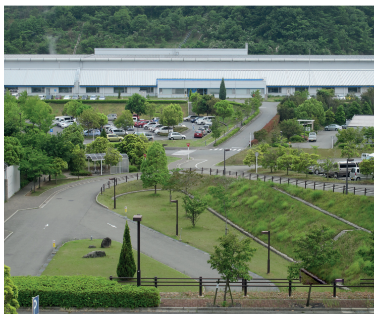
SPring8 - the world's largest third-generation synchrotron radiation facility located in Hyogo, Japan
